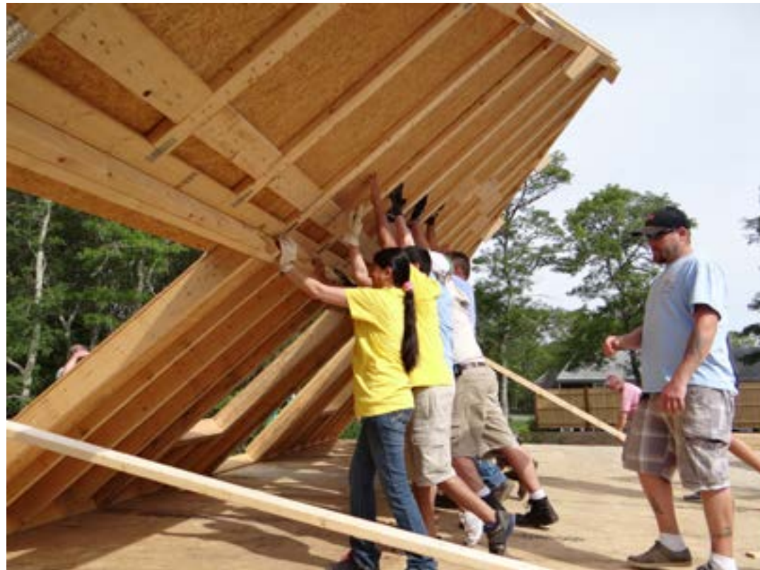
Volunteers raise a wall on Oak Street in Harwich
