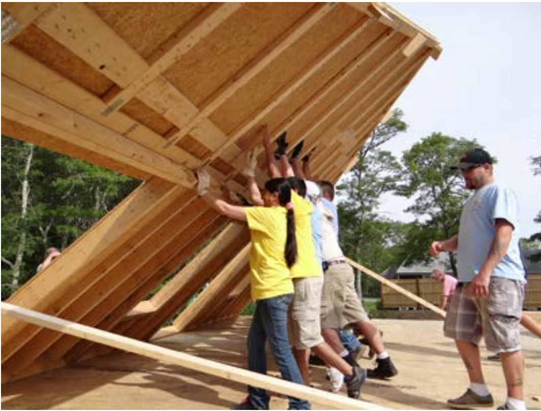
Volunteers raise a wall on Oak Street in Harwich
